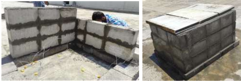
Trombe Wall Construction
