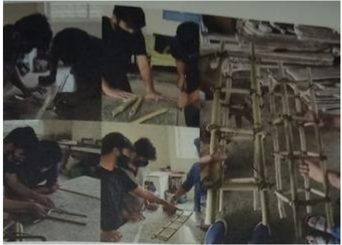
Making of bamboo Reinforcement
